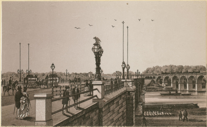
GIRARD AVENUE BRIDGE.
