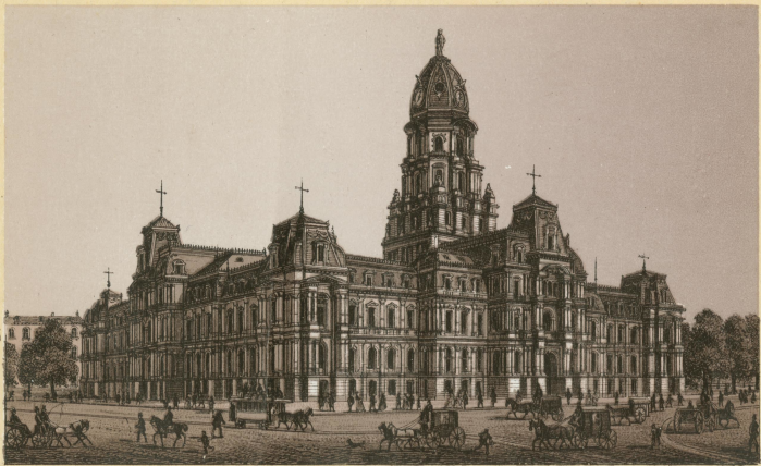
THE PUBLIC BUILDINGS.
