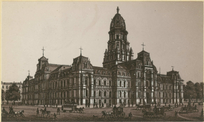
THE PUBLIC BUILDINGS.
