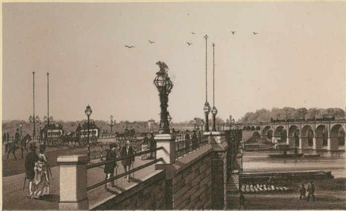
GIRARD AVENUE BRIDGE.
