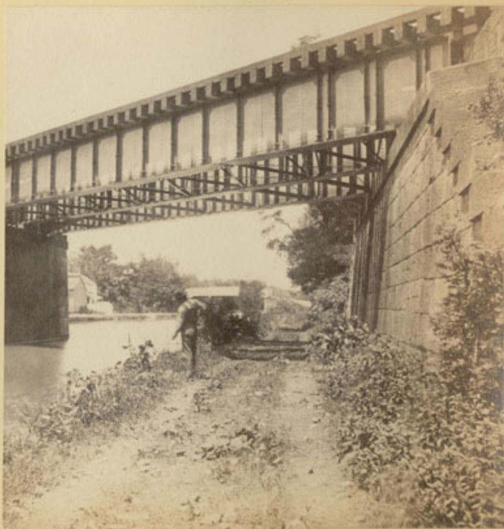
Bridge over Canal Rockville
