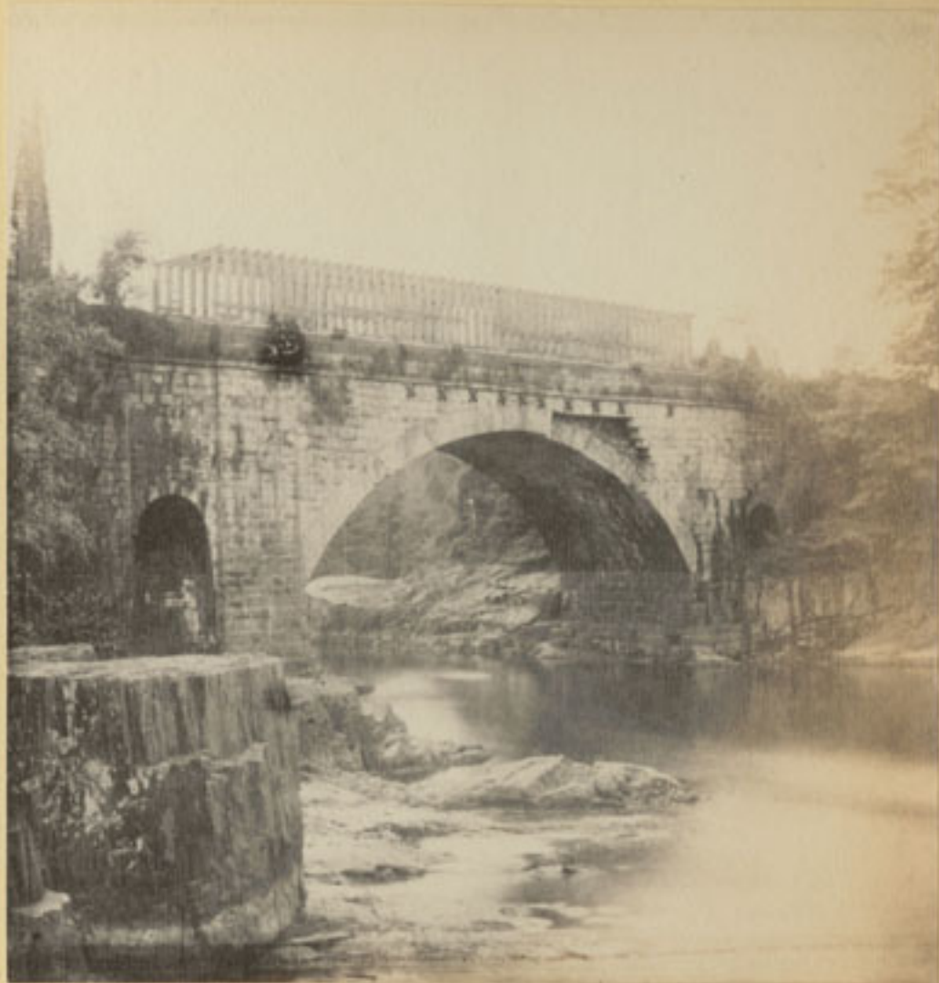
Little Falls Aqueduct
