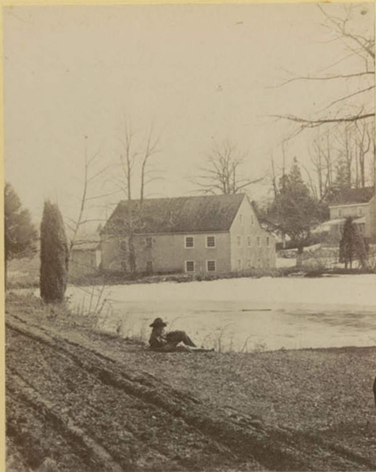
65 Mill near Milestown
