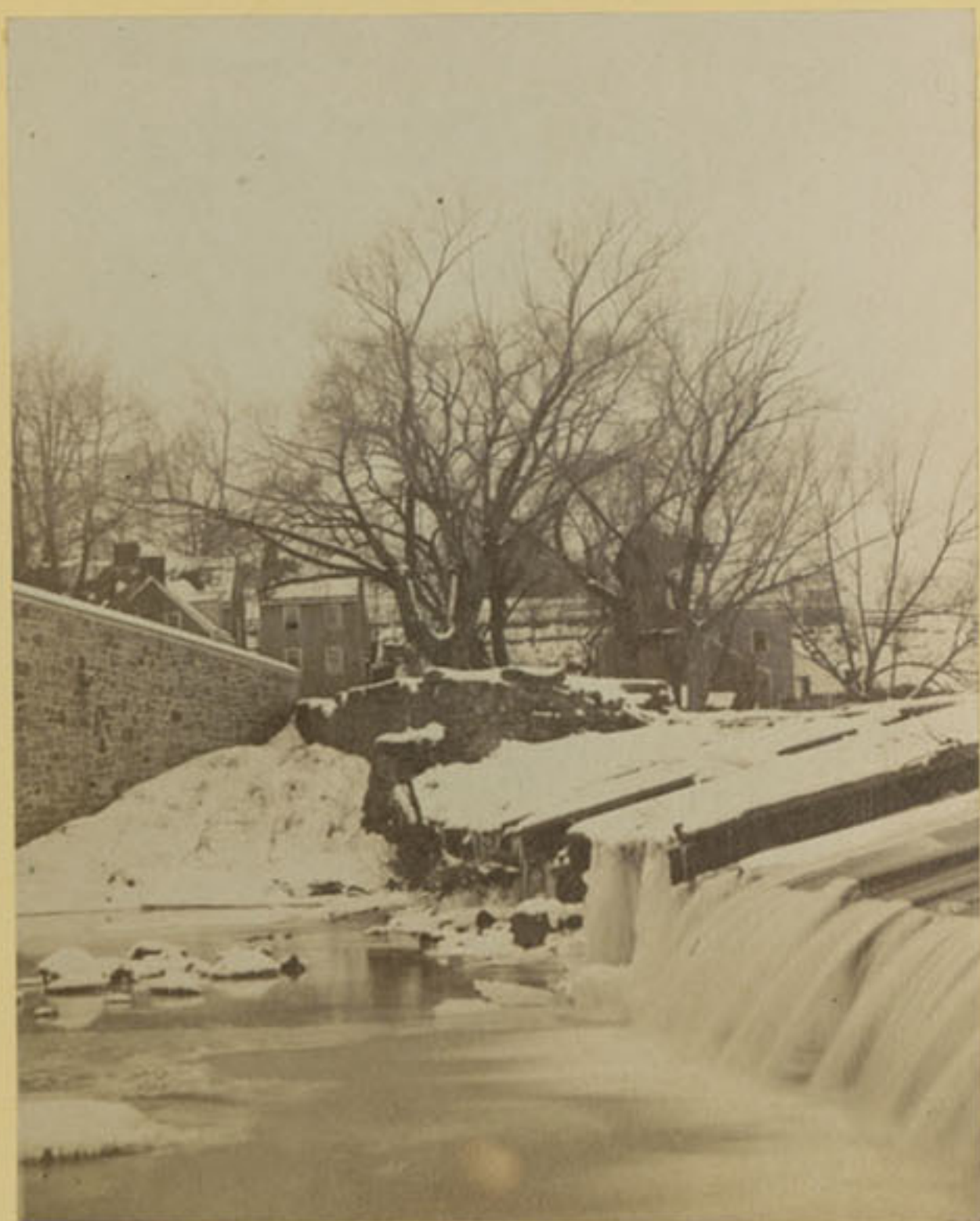
66 Dam Breast at Crescentville
