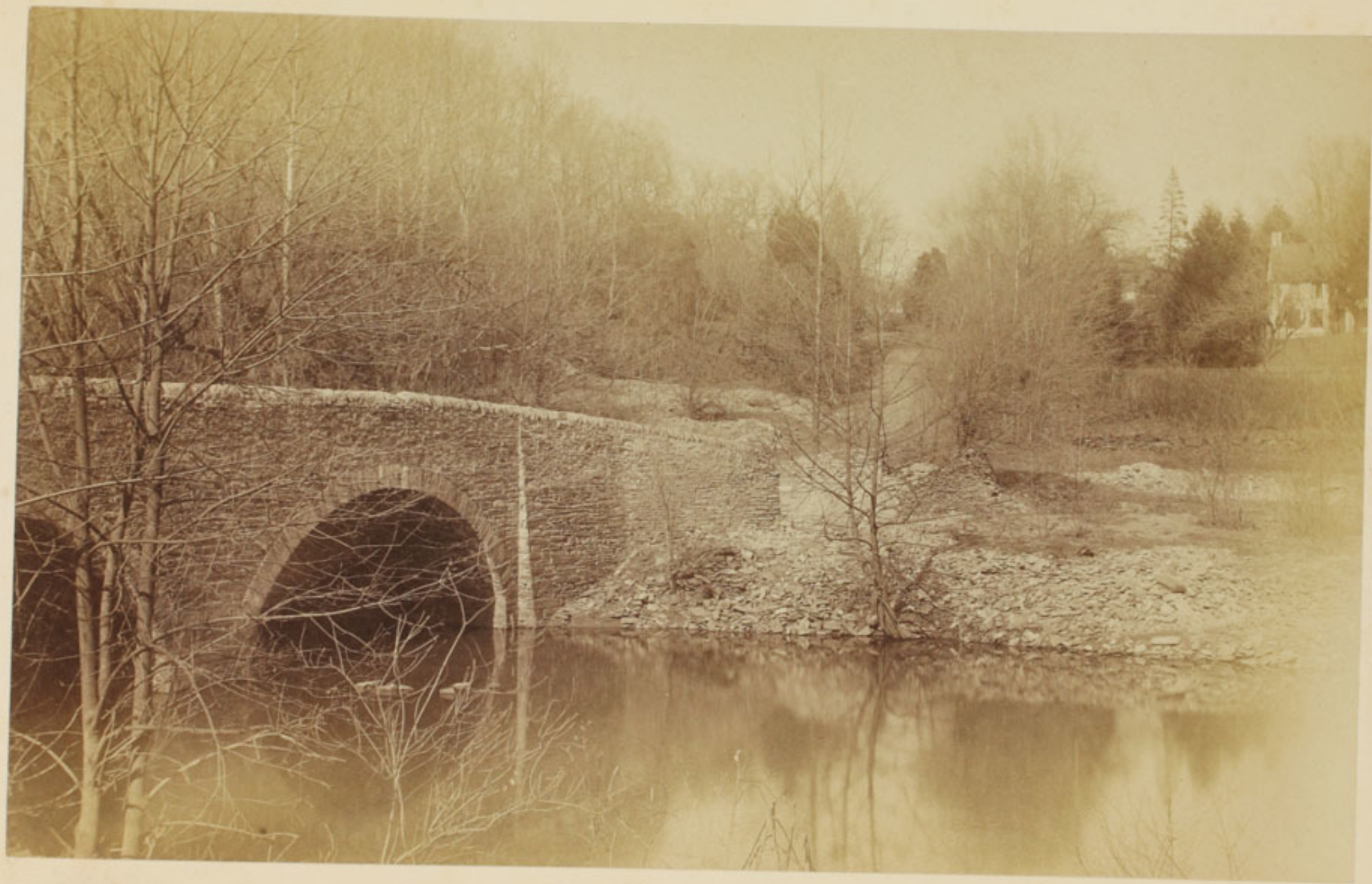
THORPS LANE BRIDGE Wissahickon
