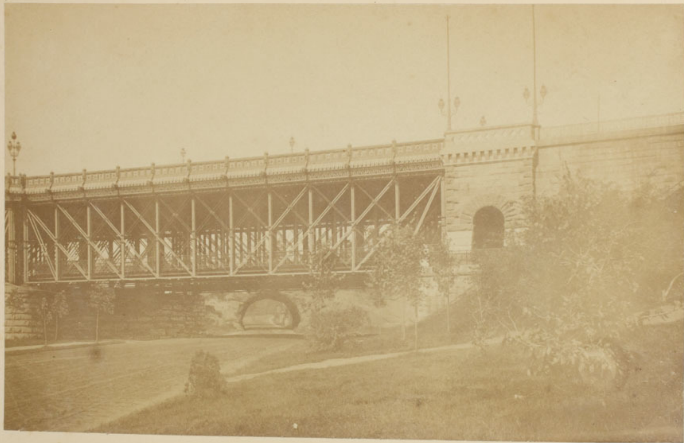
Girard Ave. Bridge and Tunnel.
