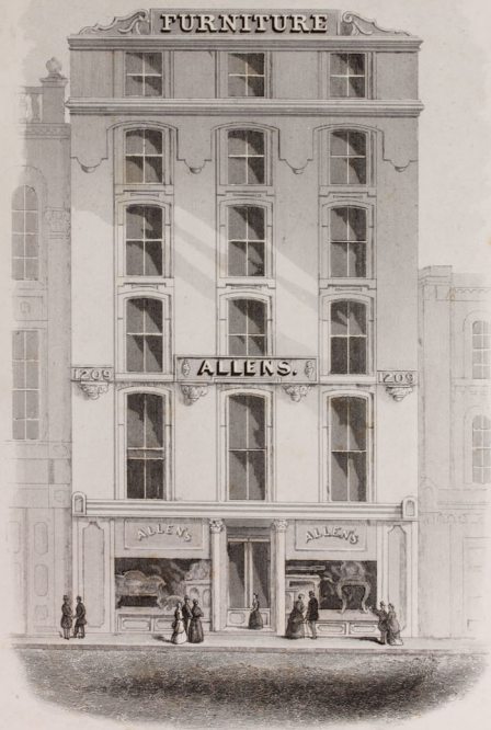
Allen's Furniture Warehouse, Philadelphia
