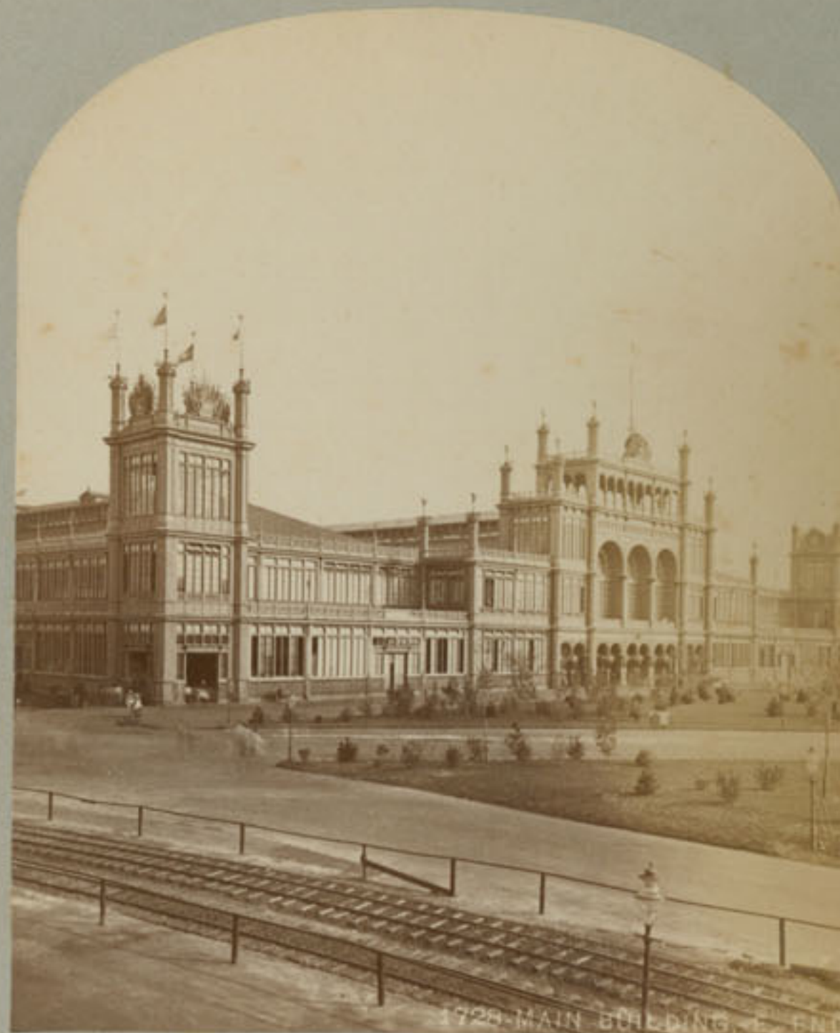
1720 MAIN BUILDING FROM EAST
