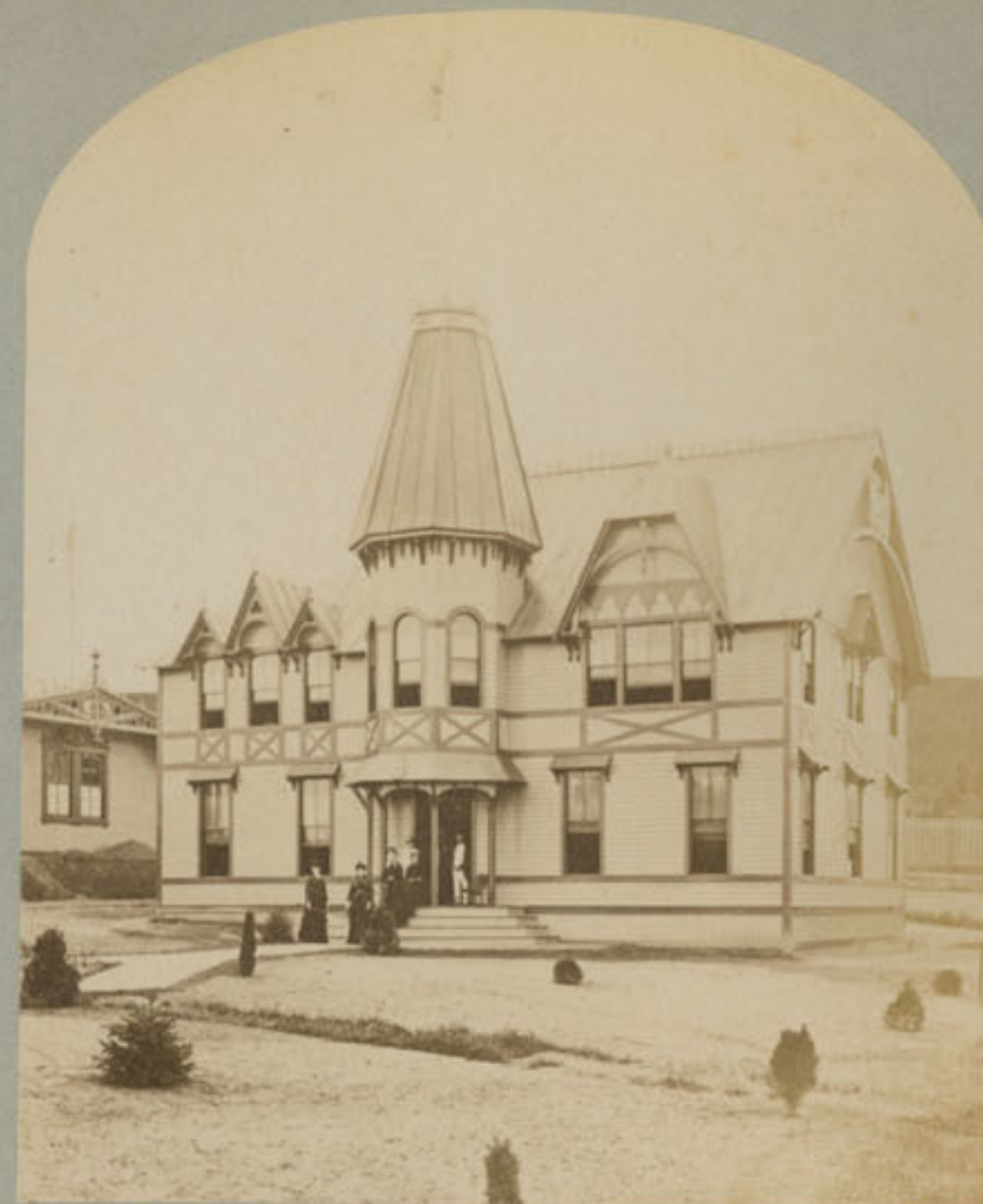
767 Delaware State Building c
