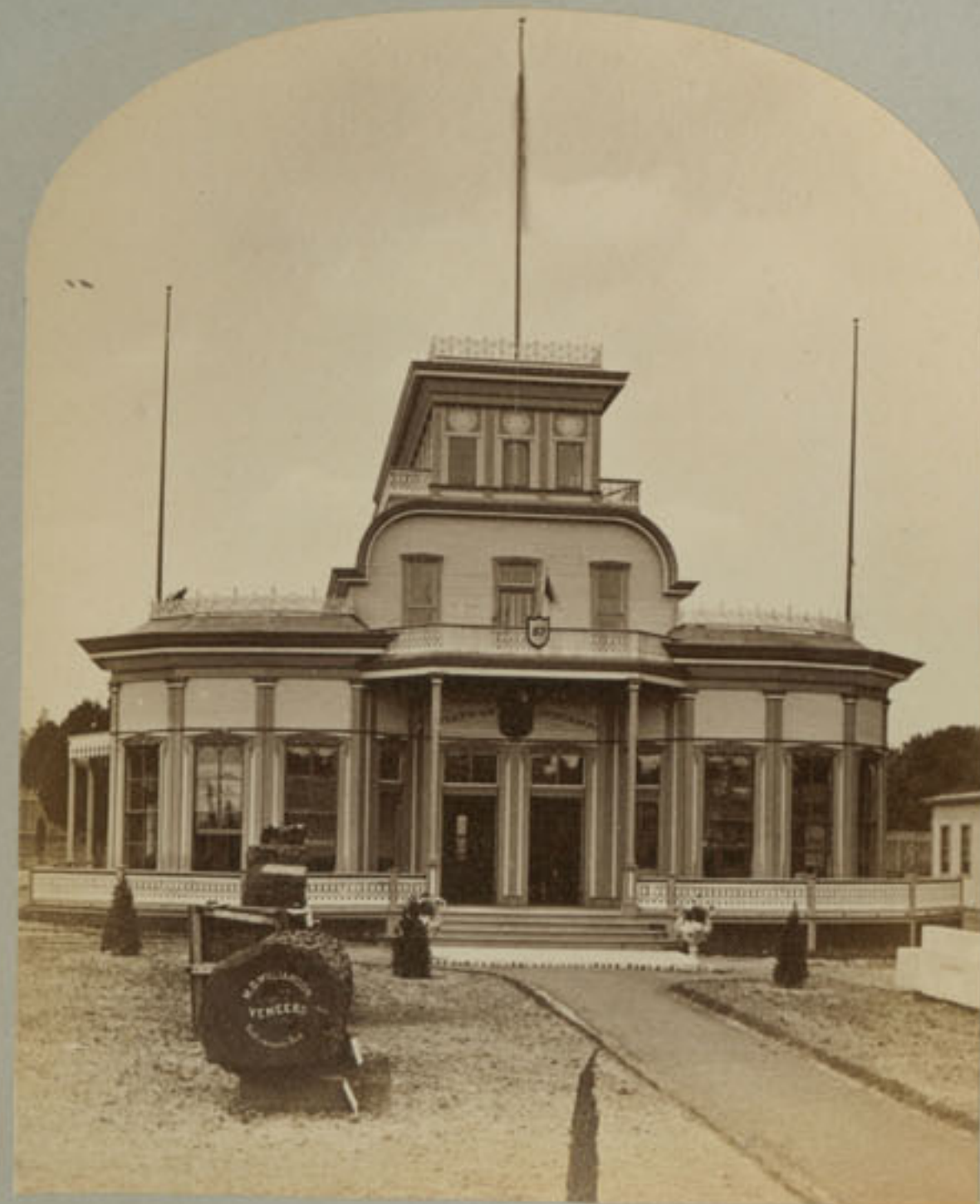
701 Indiana State Building
