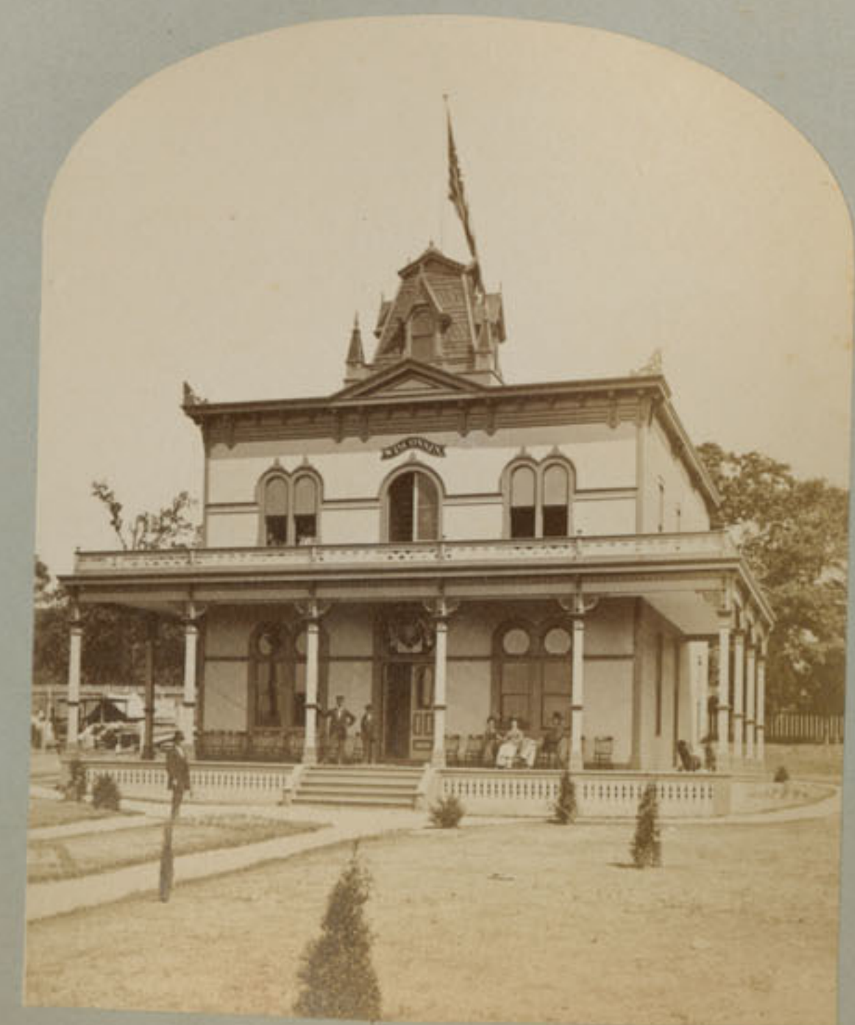
722 Wisconsin State Building
