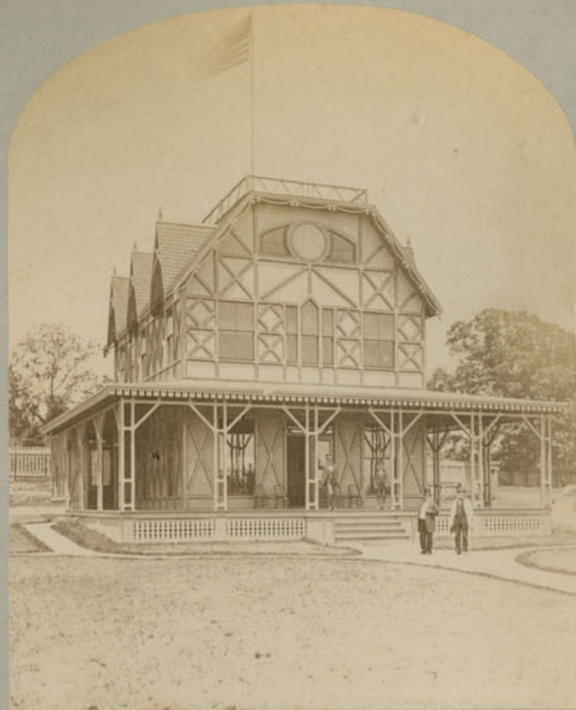
704 New Hampshire State Building
