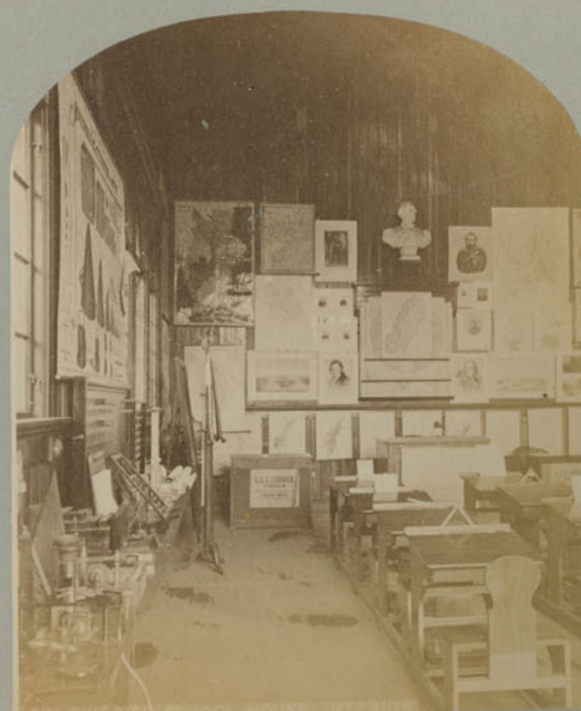
1911 SWEDISH SCHOOL HOUSE, INTERIOR
