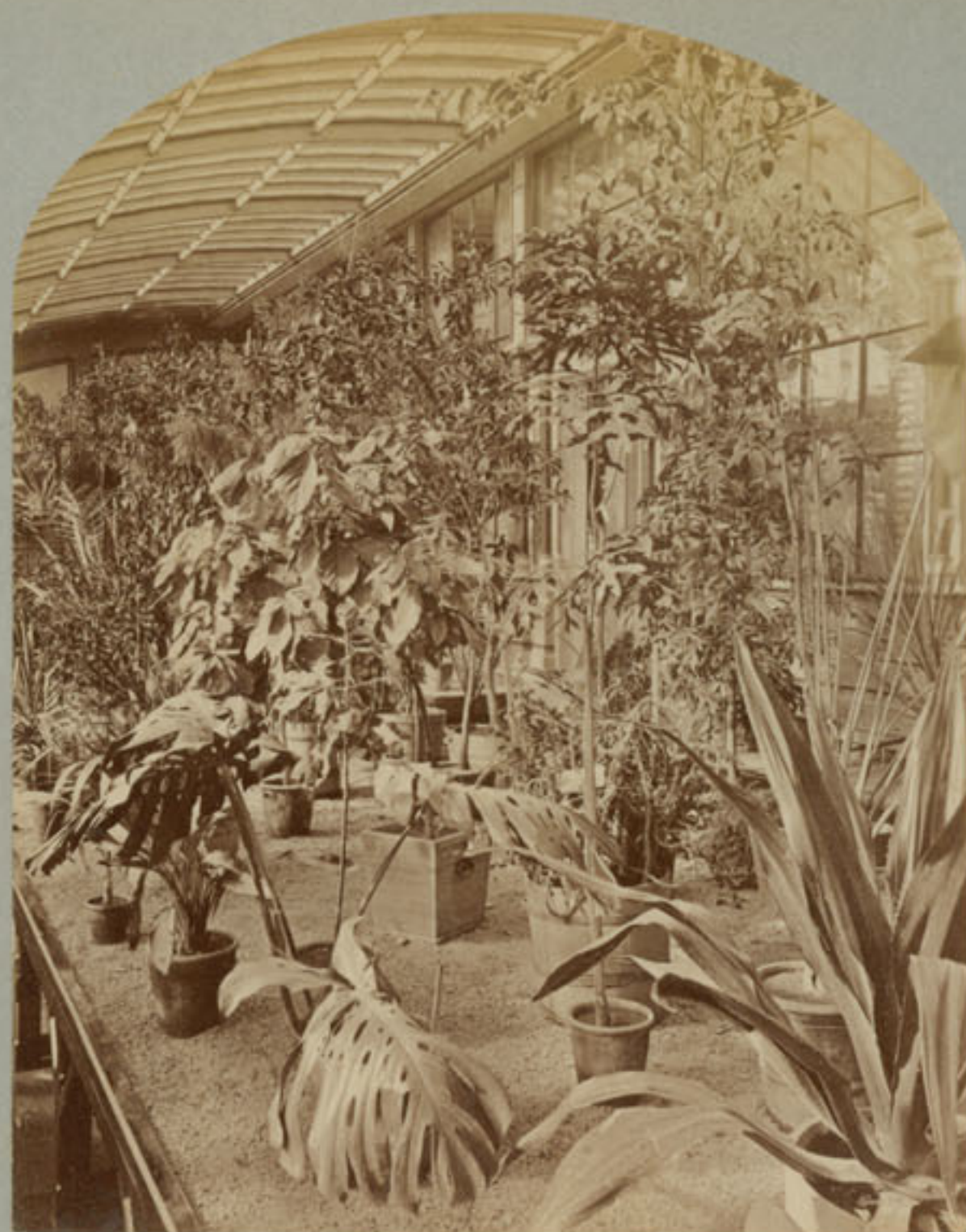
53 Horticultural Building S.E. Forcing Room
