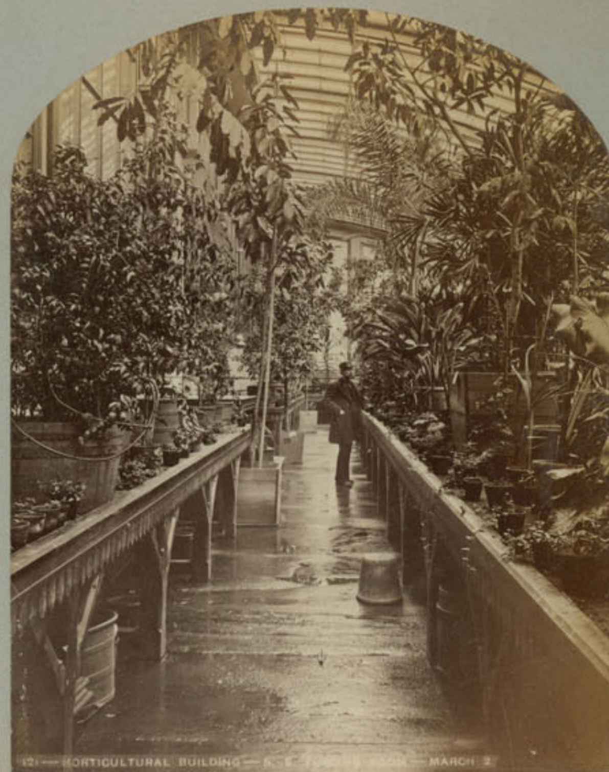
121 HORTICULTURAL BUILDING - S. E. FORCING ROOM - MARCH 2
