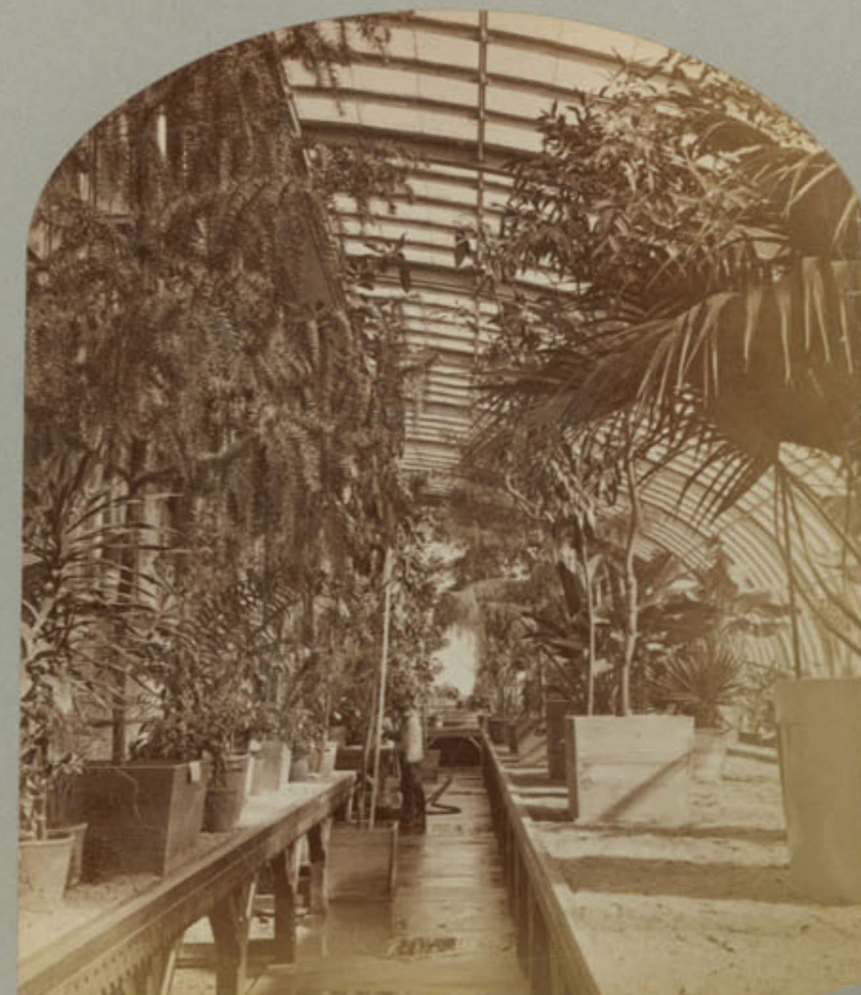
65 Horticultural Building - S.E. Forcing Room
