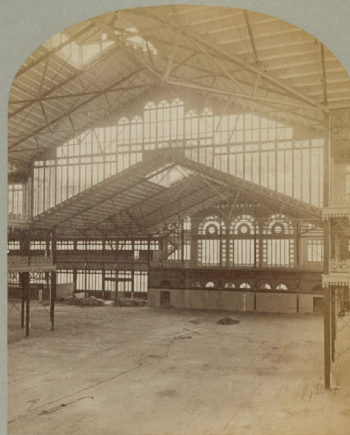
108 Main Building - Transept
