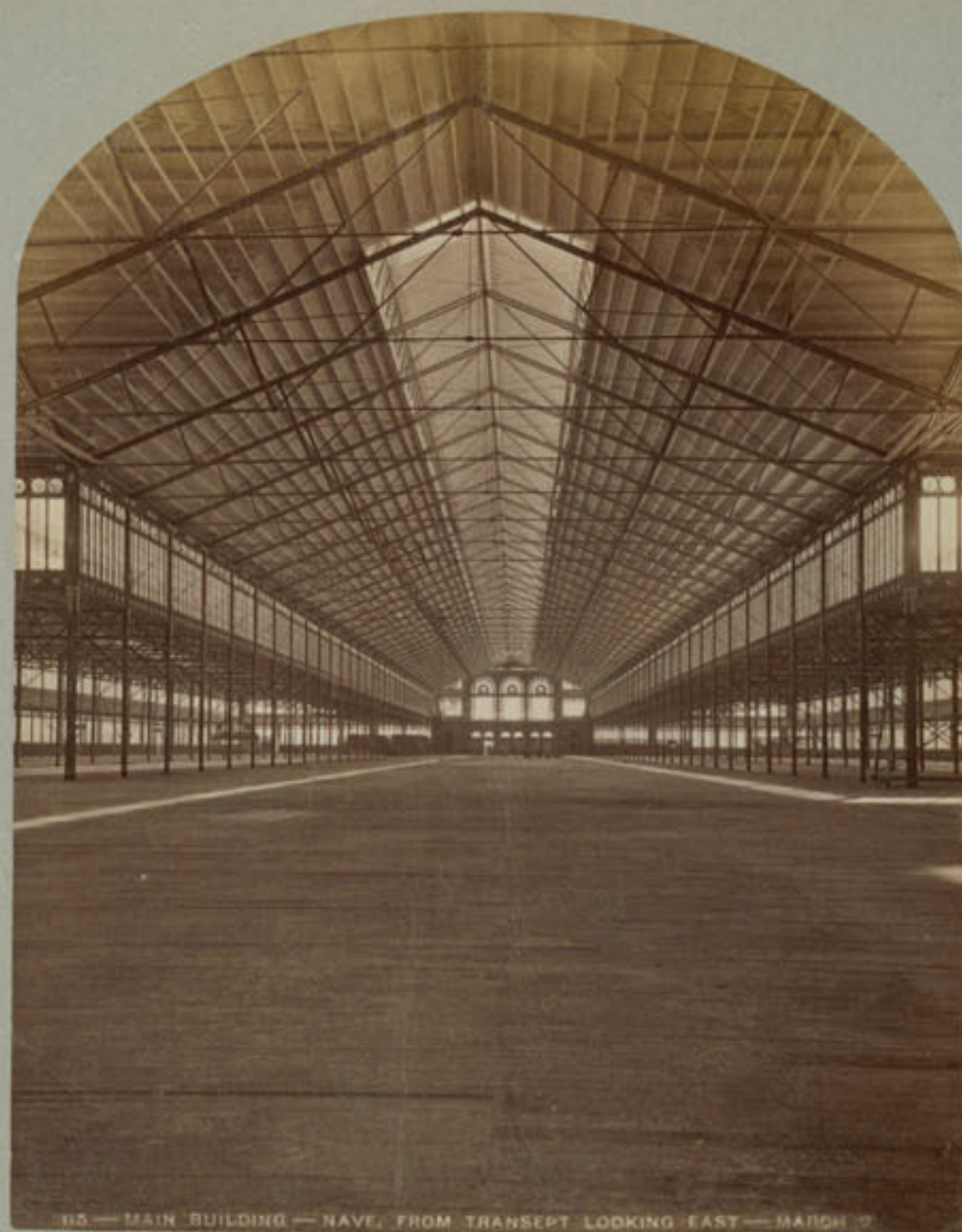
105 - MAIN BUILDING - NAVE, FROM TRANSEPT LOOKING EAST - MARCH 2
