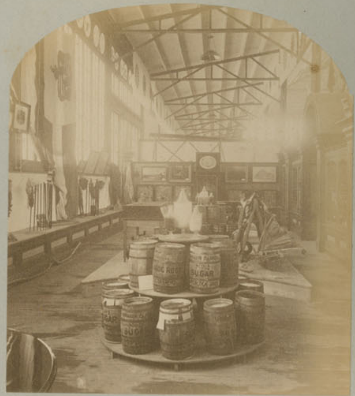
791 Hawaiian Exhibit - Main Building
