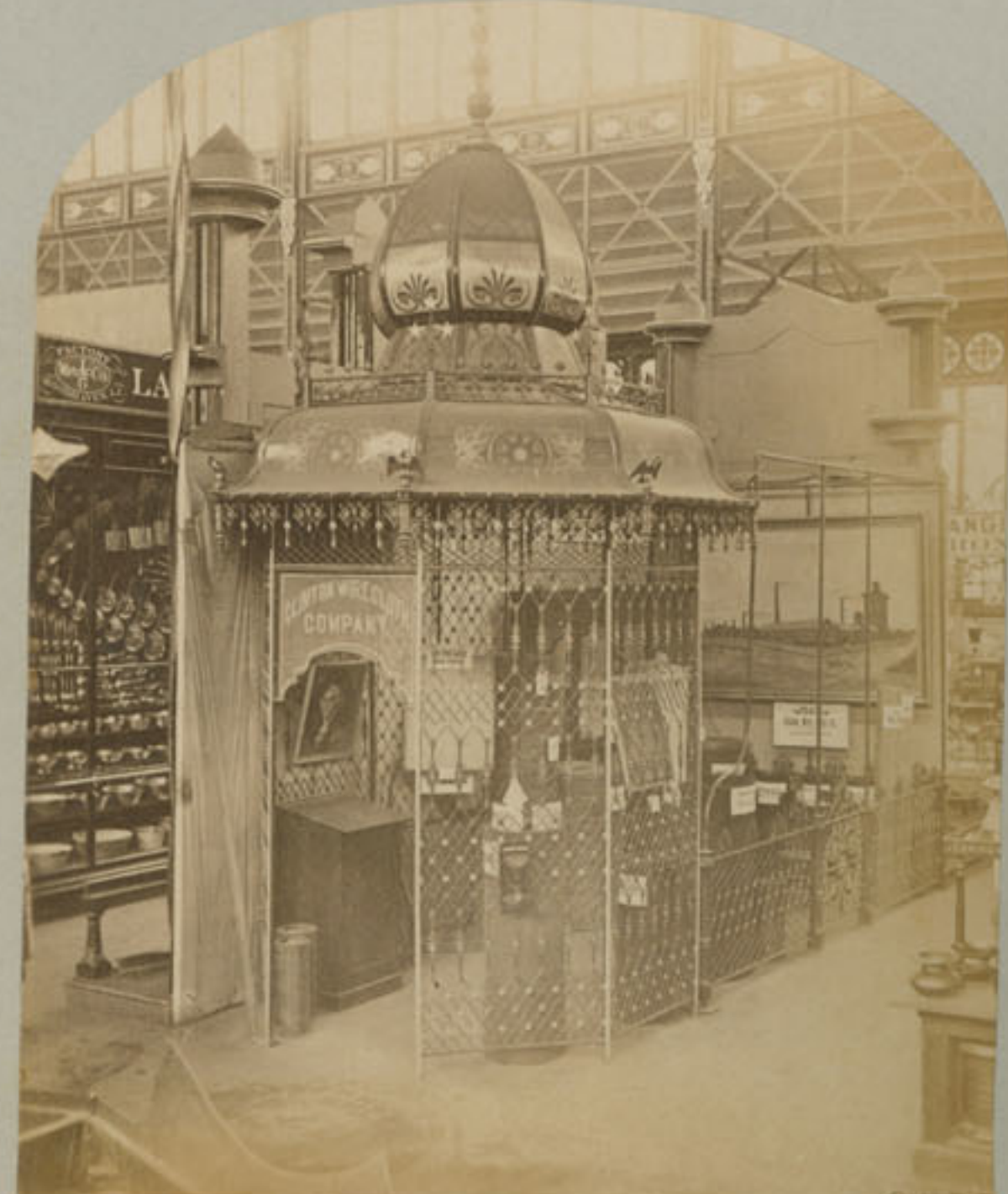
2472 - Clinton Wire Cloth Exhibit - Main Building
