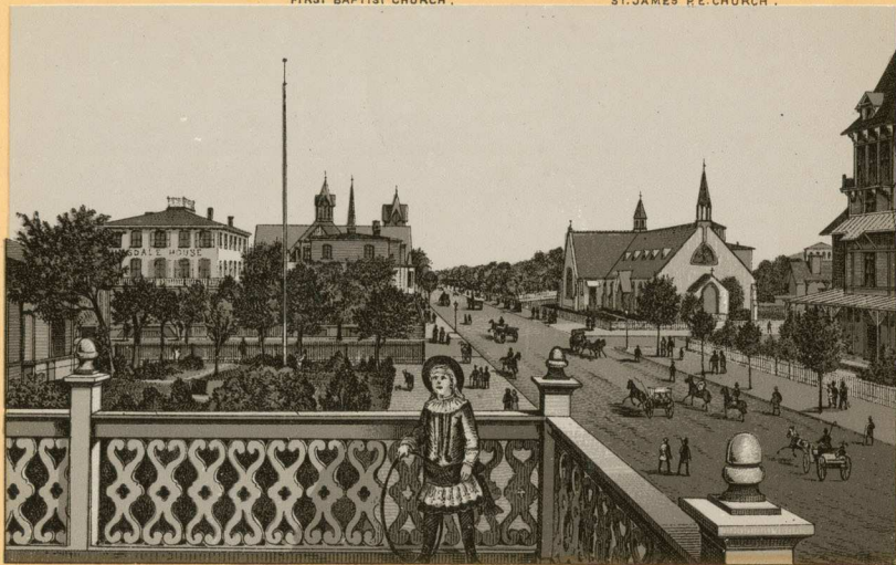
INTERSECTION OF PACIFIC AND NORTH CAROLINA AVENUES.
