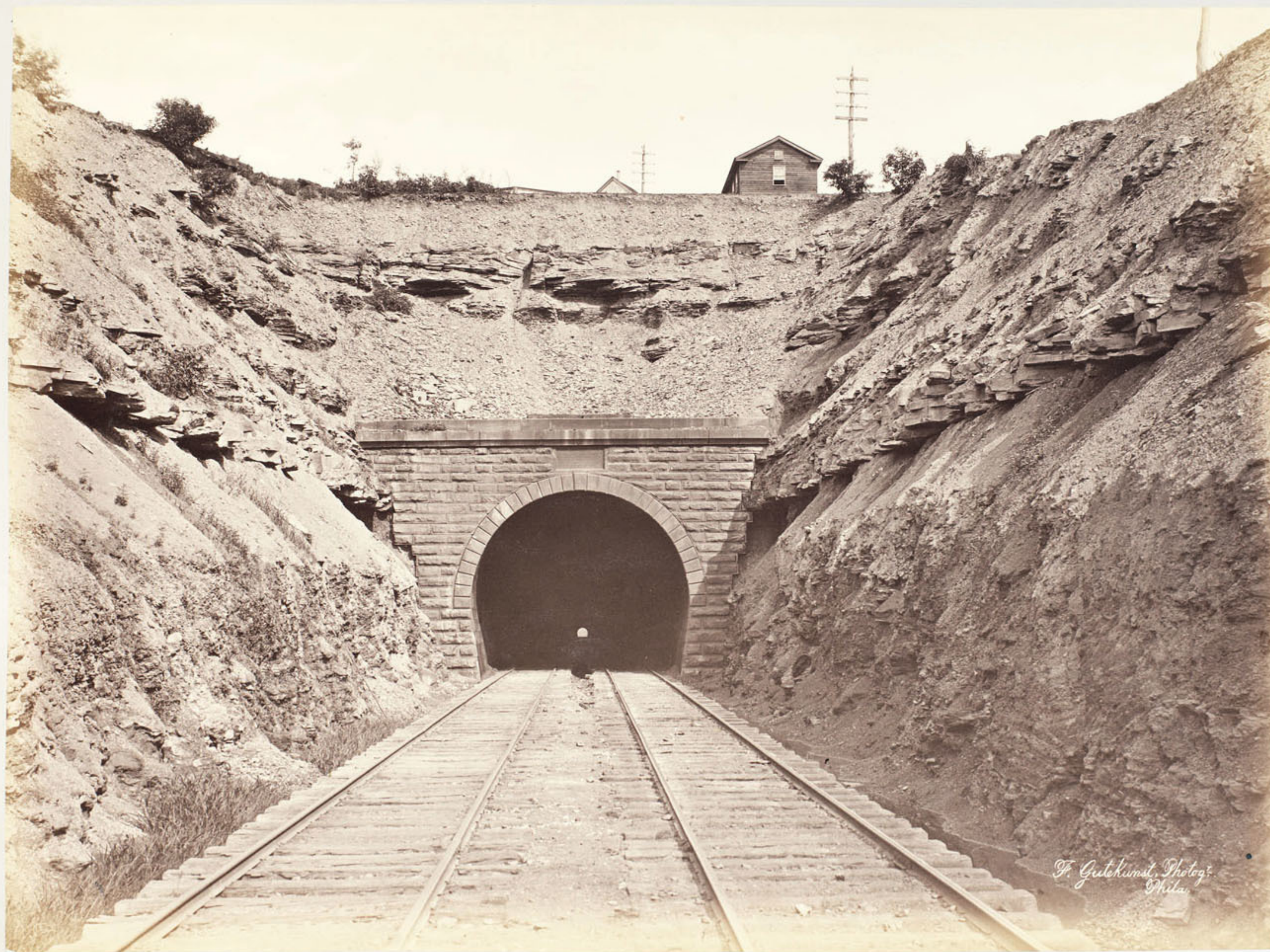
No 82 Allegheny Tunnel.
